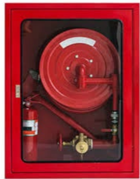
Fire hose reels
